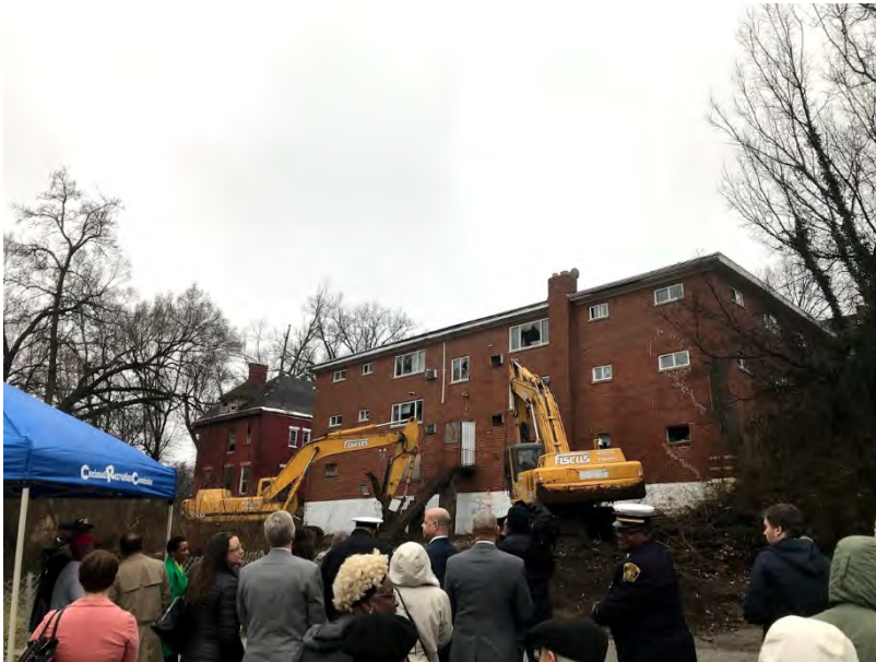
Home on Hallwood demolished by Landbank
